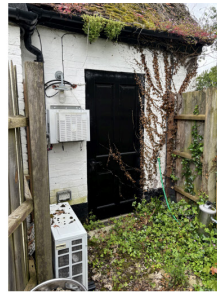
EXISTING SERVICE DOOR
