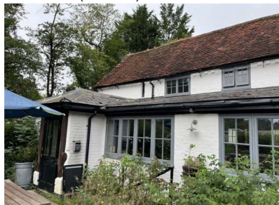
REAR (ROOF / EXISTING LEAN TO)
