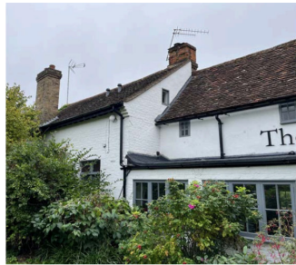
FRONT (ROOF DETAIL)
