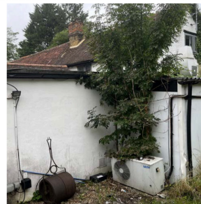
SIDE, NORTH ELEVATION (MECHANICAL PLANT)
